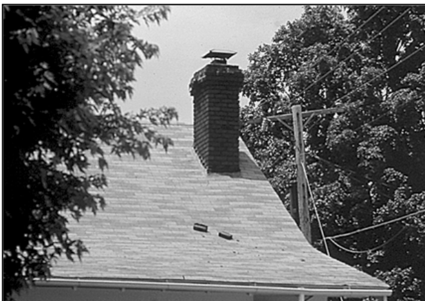
Typical minor damage (Modified Mercalli Intensity VI to VII) from Lawrenceville, Illinois M 5.0 earthquake. Bricks thrown from Chimney and diagonal masonry cracks in church tower.
