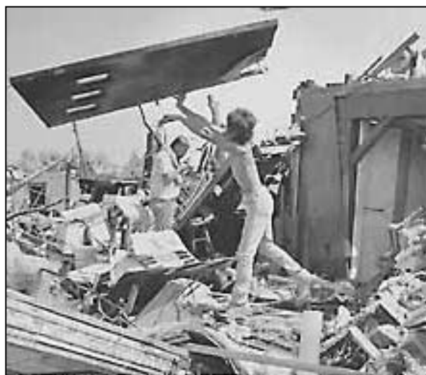
Tornado Damage in Plainfield
