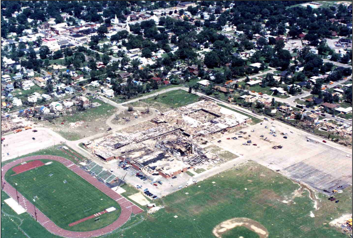
Damaged Plainfield High School
