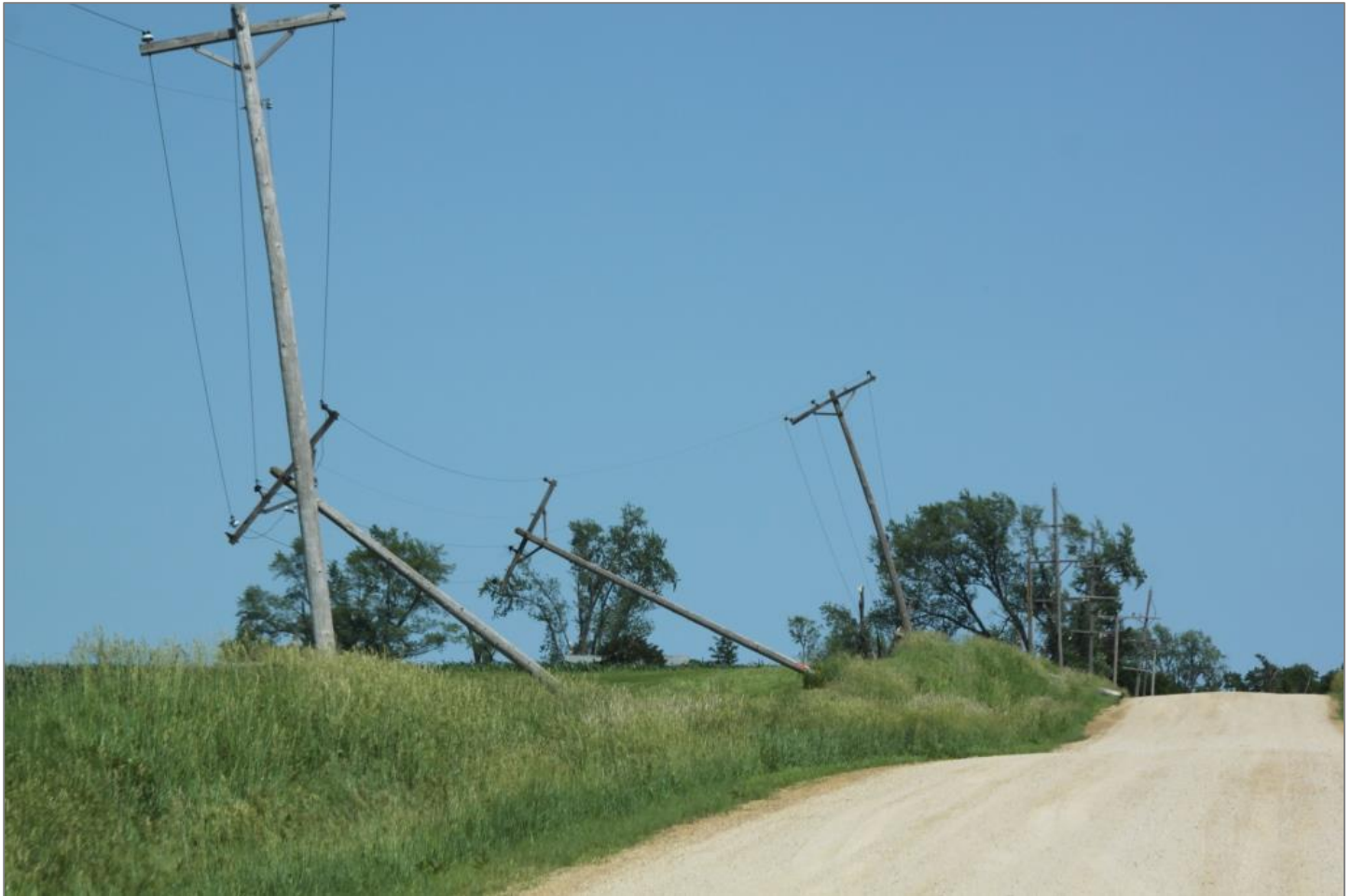
Photo 1: June 2014 damage to utility poles and trees in rural Lena resulting from straight-line wind and microburst activity – source: SCEMA
