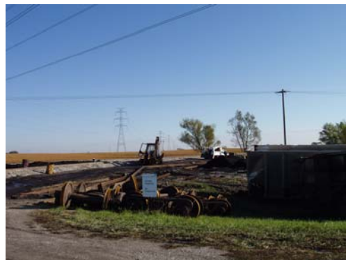
Coal car derailment at Baldwin Plant (derailment and cleanup did not impact residents or businesses), October 2004
