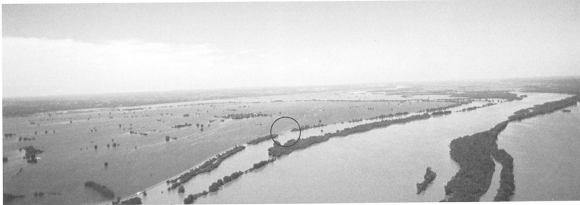
Kaskaskia Island looking north. Circled area shows broken levee.
