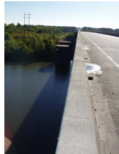
Bulkheads protect the piers of the State Route 154 Bridge at the Kaskaskia River.
