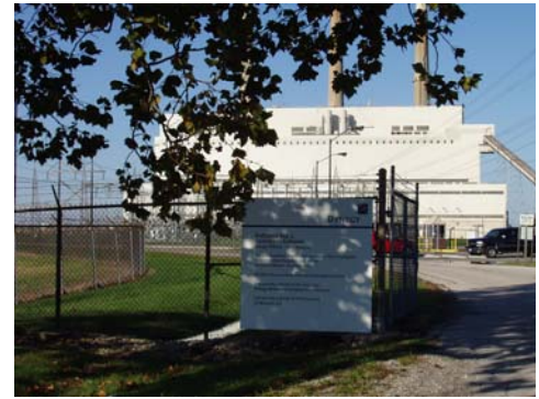
Dynergy Power Plant near Baldwin
