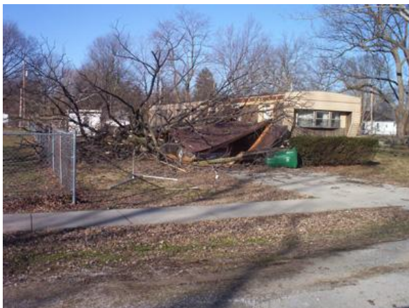
File: Winter2_Jan_2008 Date: January 29, 2008 Description: Storm damage in Mounds, IL on January 29, 2008.. Source: http://community.wpsdtv.com/photos/storm_photos/category1798/picture2461338.aspx
