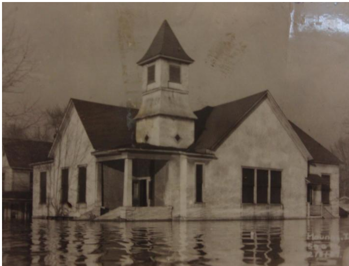
File: Flood5_Jan_1937 Date: January, 1937 Description: Old Methodist Church Source: Mounds Public Library, Mounds, IL
