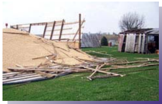
Damage sustained to a grain bin in rural Ogle County from a thunderstorm accompanied by high winds.
