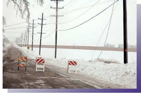
Ice accumulations from the December 24 th , 2009 ice storm downed communication and power lines.
