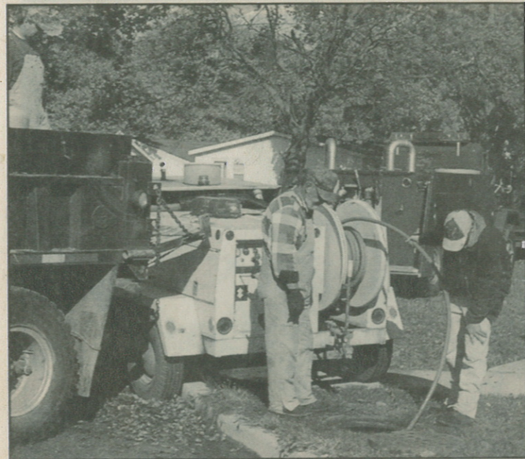
Dennis Kates and Keith Rickman keep an eye on the cable that operates the root saw blade which is being used at the intersection of State and North High Street in the first phase of the Lovington water drainage project. Standing in the back of the truck is Dennis Coslow.
