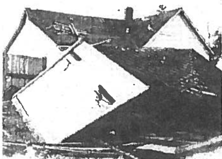
West view of Lloyd Lilly place east of Allenville. In the foreground is the garage. The walls were torn out and the roof rested on the car, which was not badly damaged.
