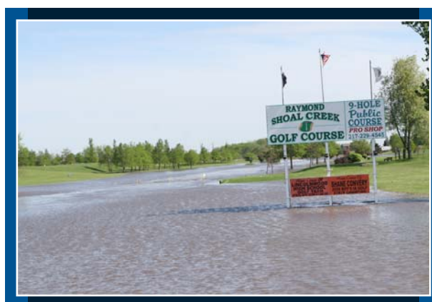
The West Fork Shoal Creek has overflowed its banks on several occasion, flood this golf course near Raymond's wastewater treatment facility.
