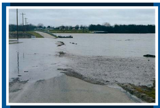
During the December 28, 2015 flash flood event, Glenn Shoals Lake overtopped Glenn Shoals Drive as the emergency spillway was utilized to handle the excess water.
