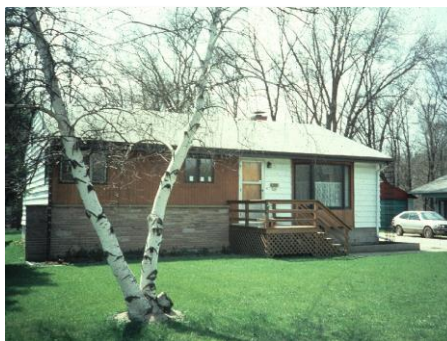
Home elevated two foot above the base flood elevation
