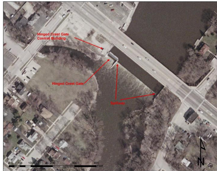
Figure 2-22 Plan View of Stratton Lock and Dam
