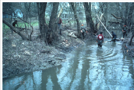
A regular inspection and maintenance program can remove debris before it becomes an obstruction to stream flows.
