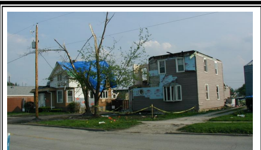
Tornado damage to residences Utica, Illinois, 2004
