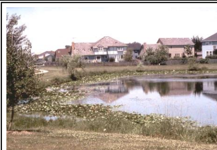
Storage ponds manage the increased runoff from new developments.
