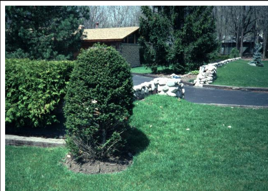
This low floodwall on the Des Plaines River has landscaping to minimize the adverse impact on the property's appearance.
