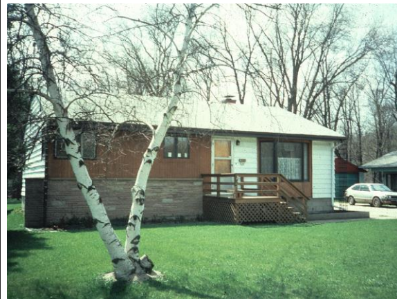
This house was elevated one foot above the base flood elevation of the Des Plaines River.
