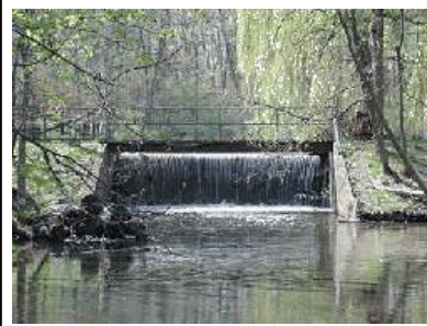
This dam on Brewster Creek was removed.
