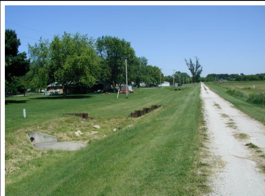
Because 30 homes were purchased after the 1996 flood, the Park View Estates levee protects some empty lots.
