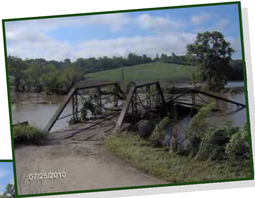
Flood Damage to Georgetown Road Bridge over Apple River northwest of Elizabeth
