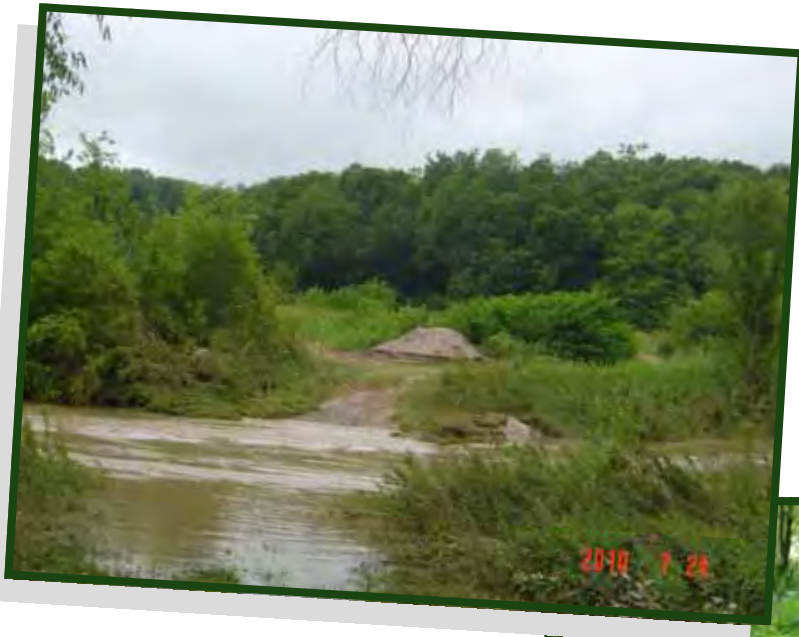
Flooding of Road to Miner Road Quarry
