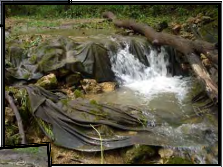
Damage to No Name Creek at Trail 6
