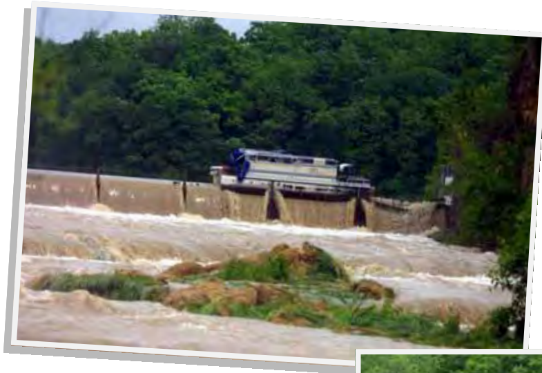
Pontoon Boat Caught on Spillway
