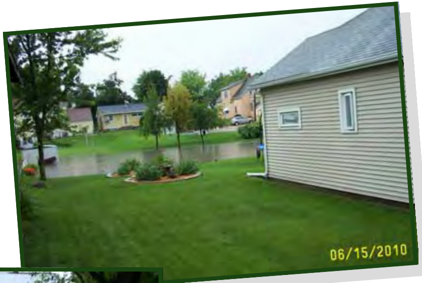
Flooding in Residential Neighborhood
