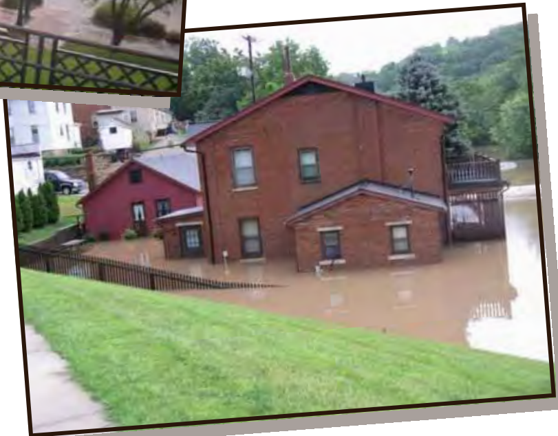
Hughlett Branch overflows its banks, flooding Meeker and Claude Streets
