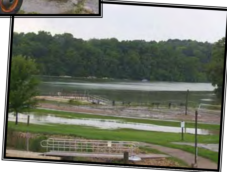
Marina Beach Flooding
