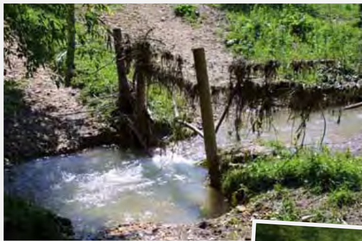
Debris Line from Flooding on Trail
