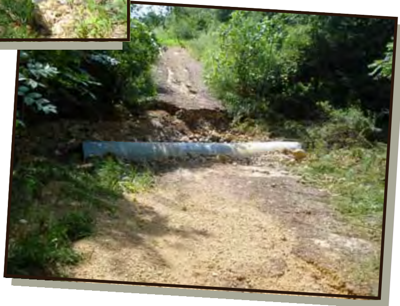
Trail washout at Powderhorn Gap
