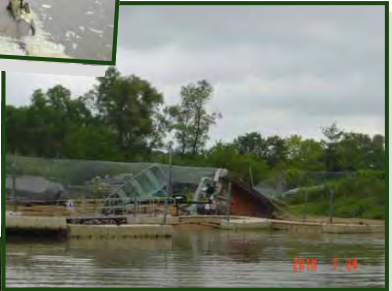
Boat Pen Damage
