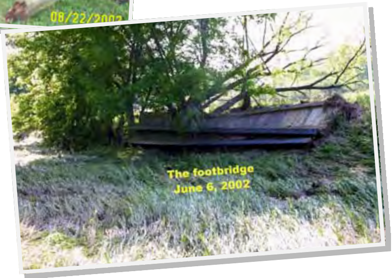
Footbridge Across Small Pox Creek at Trail 4
