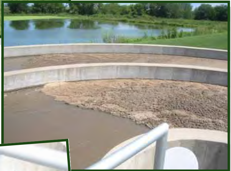
Flooding at Wastewater Treatment Facility
