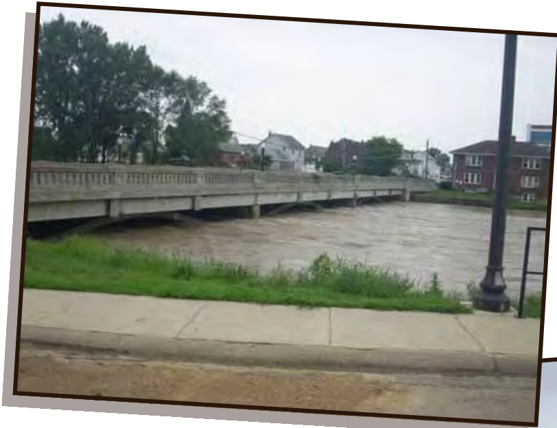
Water laps at the underside of the Illinois Rte. 84 bridge over the Apple River
