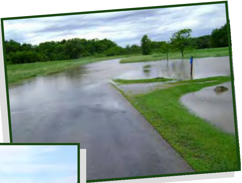
Flooding on Marina Drive
