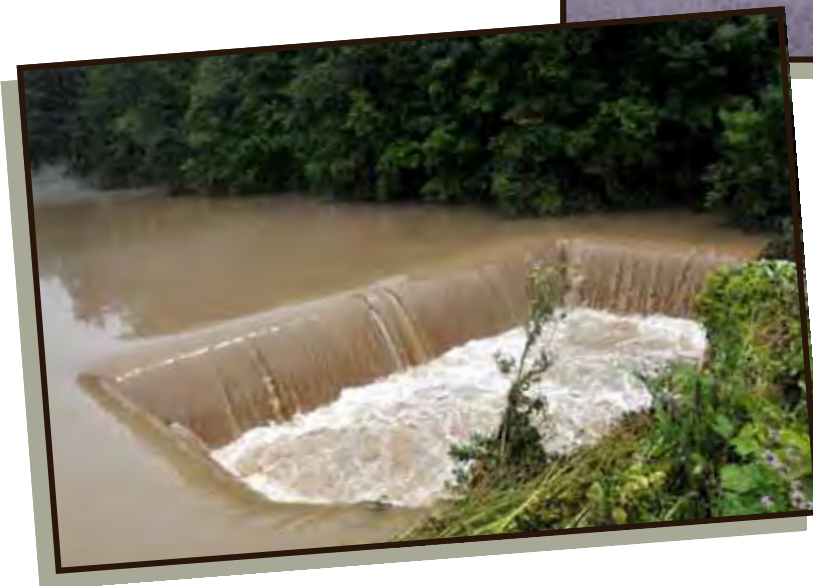
Sedimentation control weir at Territory Drive
