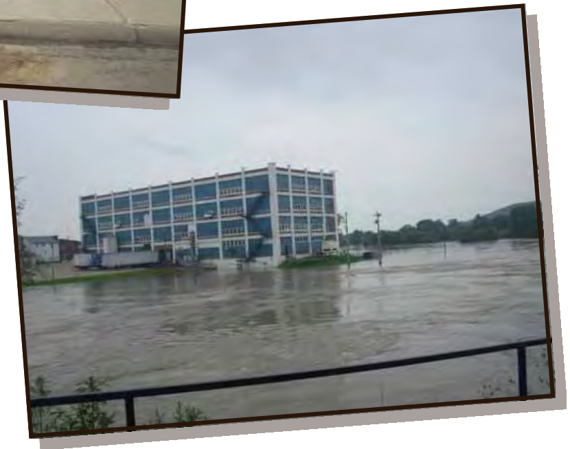
Flood waters from the Apple River partially surround the Invensys Appliance Control Building
