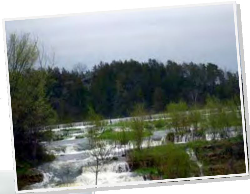
Spillway from Thunder Bay Road
