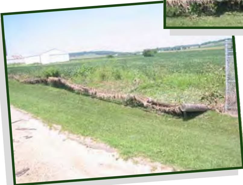
Fence Damage Caused by Flooding adjacent to the Wastewater Treatment Facility
