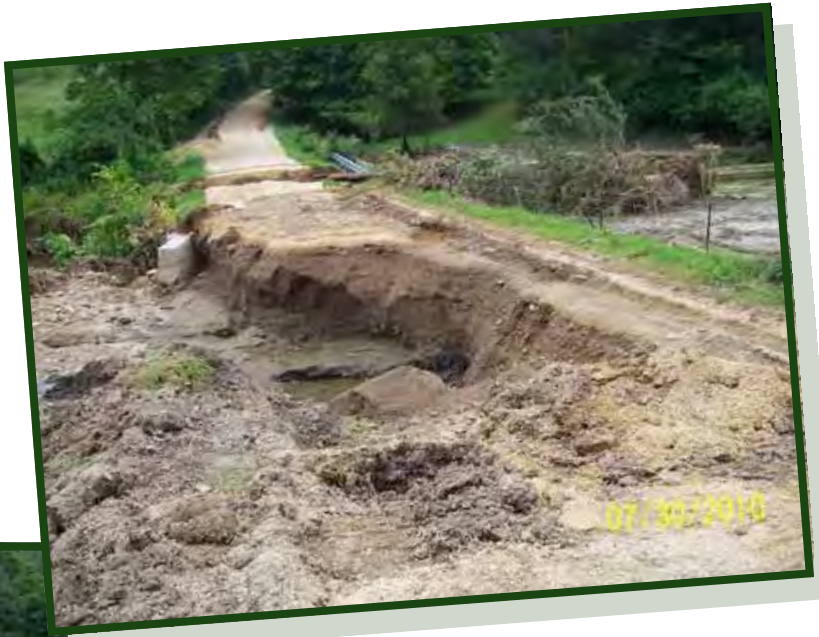
Flood Damage to Upman Road in Rush Township
