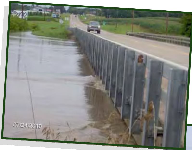
US Route 20 bridge over the Apple River west of Elizabeth
