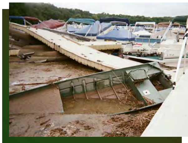
Boat and dock damage sustained at The Galena Territory marina during the August 9, 2009 flash flood event.
