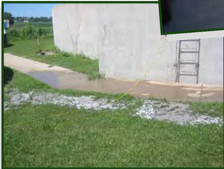
Flooding at Wastewater Treatment Facility
