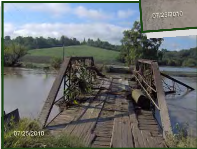
Flood Damage to Georgetown Road Bridge over Apple River northwest of Elizabeth
