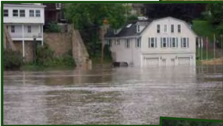
The Galena River overflowed its banks, flooding South Main Street just south of the flood gates to the downtown area
