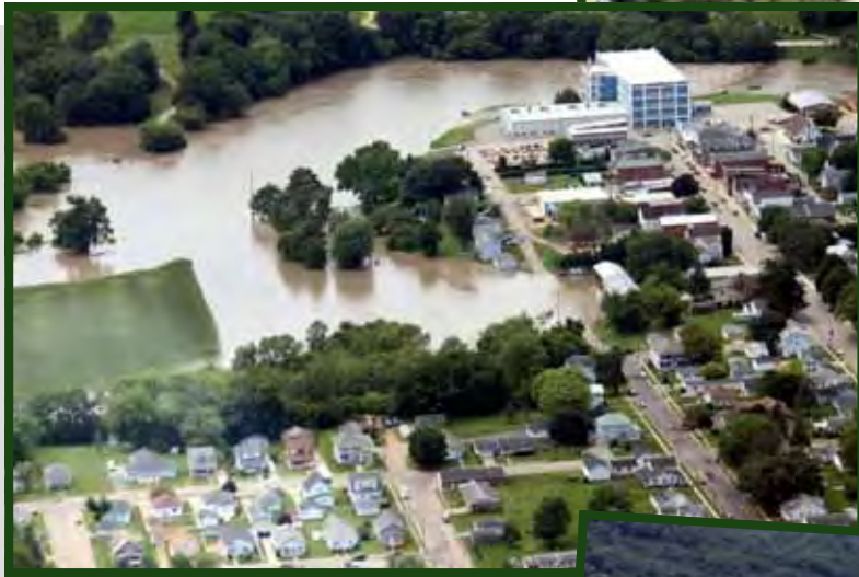
The Apple River overflowed its banks, flooding portions of Hanover including the sewage treatment lagoon on the south side of the Village (aerial photographs taken looking west)
