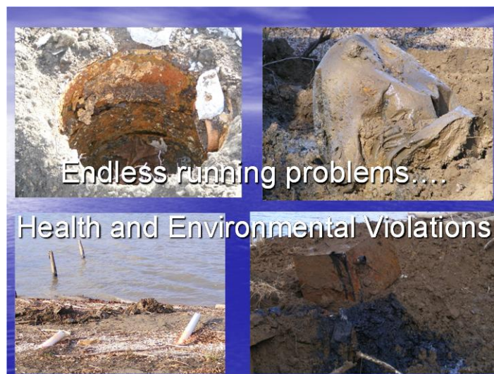
Figure 2.2.6 Original Septic Systems Removed
