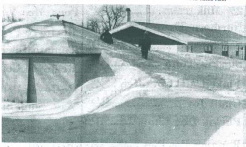
Figure 13. The blizzard of 1978 caused drifts of several feet in height and shut down many communities across the Midwest for several days.
