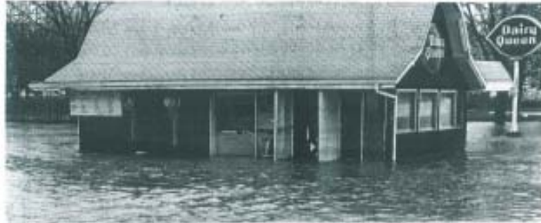
Figure 7. This Dairy Queen was flooded in April, 1994 in Cissna Park. This event caused total damages of approximately $150,000.
