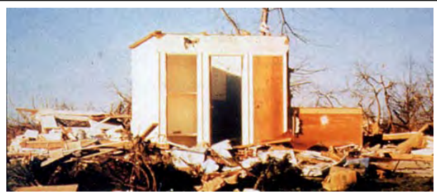
Interior rooms can be reinforced and retrofitted to be tornado “safe rooms”
