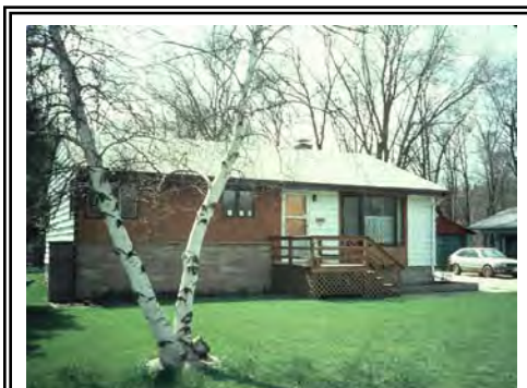
Home elevated one foot above the base flood elevation.
