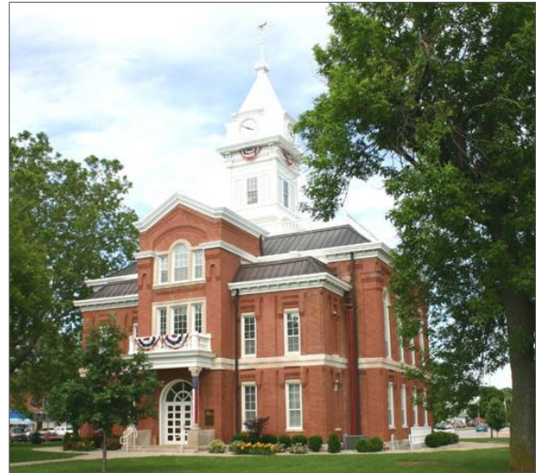
Cumberland County Courthouse, Toledo Illinois
