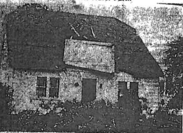
The tornado damaged the Bob Hurst farm home, two miles southeast of the Guymon farm, by twisting the porch from the house and demolishing it on the roof. Limbs from trees caused damage to the house, also. Crops in the area were leveled by the winds. A large barn and two smaller buildings on the Hurst farm were demolished. (Photo by Bertram Studio)
