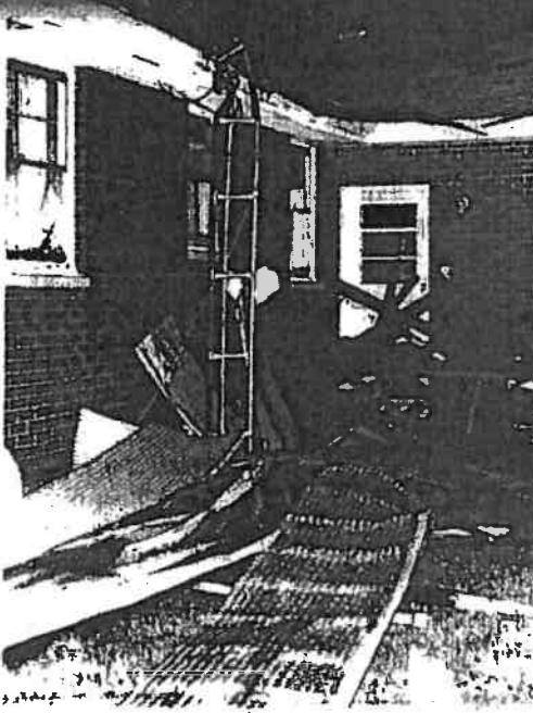
Scattered piping debris at rear of Mrs. Emery Hill residence on Lora Road.
