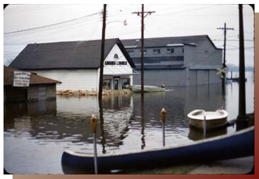
Many businesses were flooded during the 1965 Mississippi River flood.
