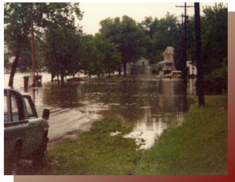
Carroll Creek floodwaters cover Mill Street in Mount Carroll during the June 13, 1981 flood.
