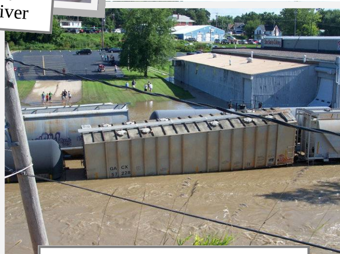
Rail lines flooded by Plum River
