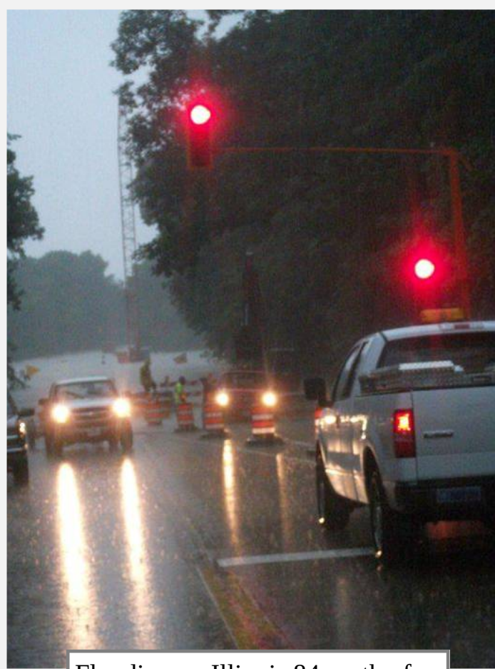
Flooding on Illinois 84 north of Savanna - in the background a crane is submerged in water
