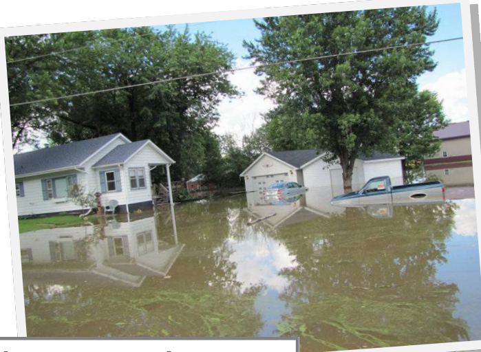
Many homes sustained serious damage as a result of the flood
