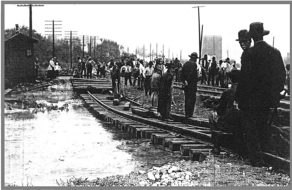
C.B. & Q. Rail Line Washout after Plum River Flood - August 11, 1911, Savanna, Ill.
