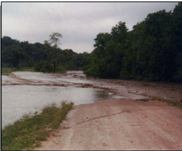
Fulrath Mill Road washed out in Fecke Flats - June 15, 1981,
