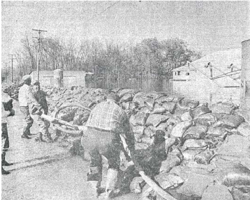
Figure 13. This sandbag wall prevented floodwaters from impacting Hardin during the 1973 flood. At the right is the Jersey County Grain Elevator.
