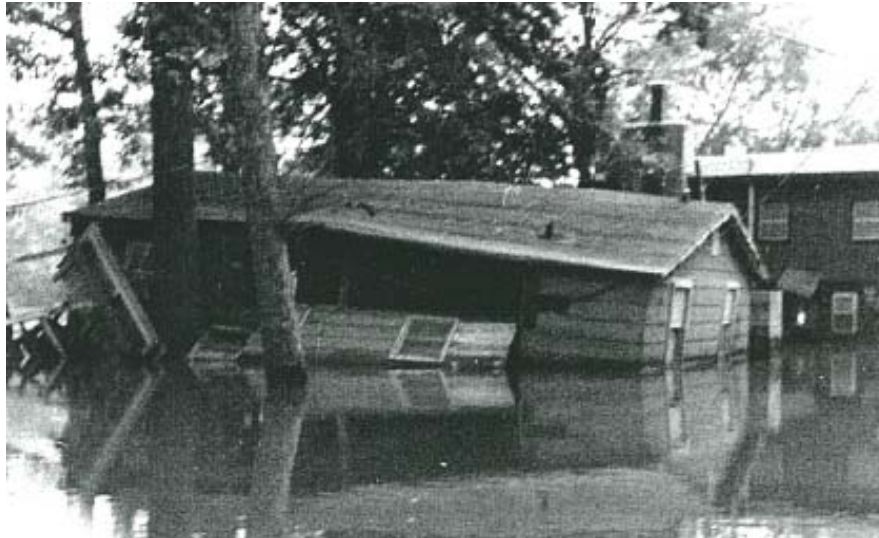
Figure 12. Flooding structurally damaged this building during the 1993 flood.
