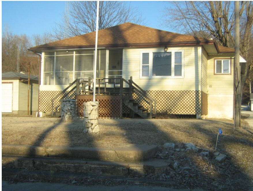
Figure 11. Home in Hamburg was raised above the base flood elevation using FEMA grant funding.
