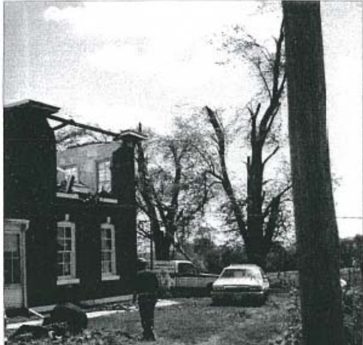
Figure 16 Home in the County was partially destroyed and the trees in the background severely damaged due to a tornado.
