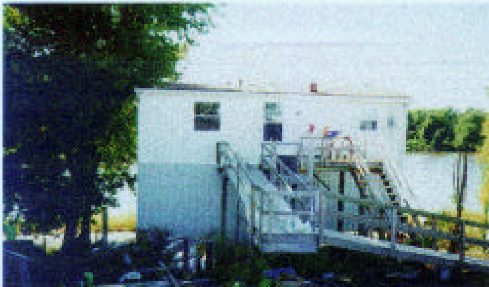
STRUCTURE AFTER ELEVATION
