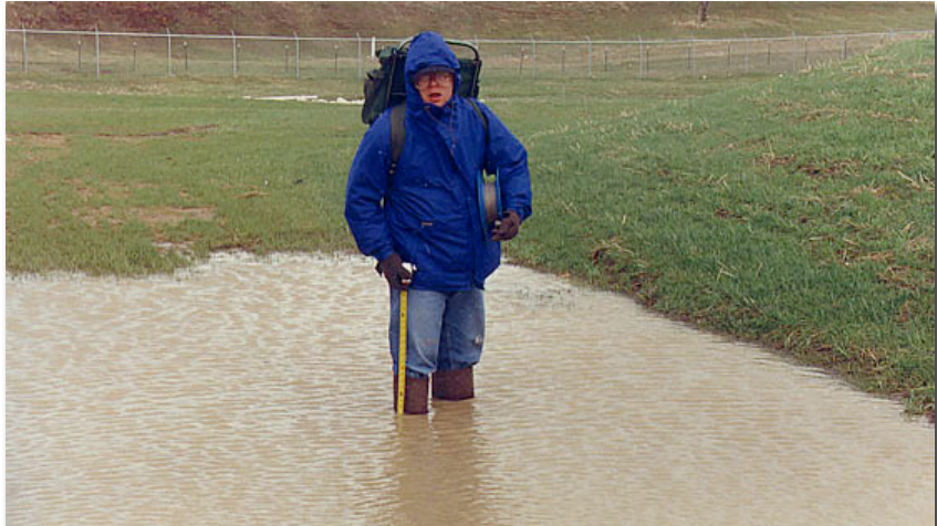
Photo 4 - State inspector standing in flooded swale at the base of a disposal trench at the Sheffield LLRW Disposal Facility (IEMA, date unknown)
