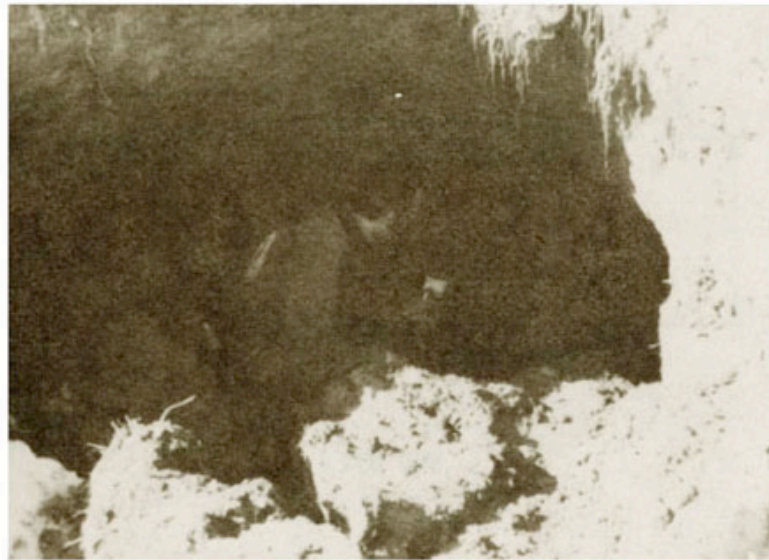
Photo 5 · Collapse holes exposed in trench surfaces after the snow melted in March 1979.
