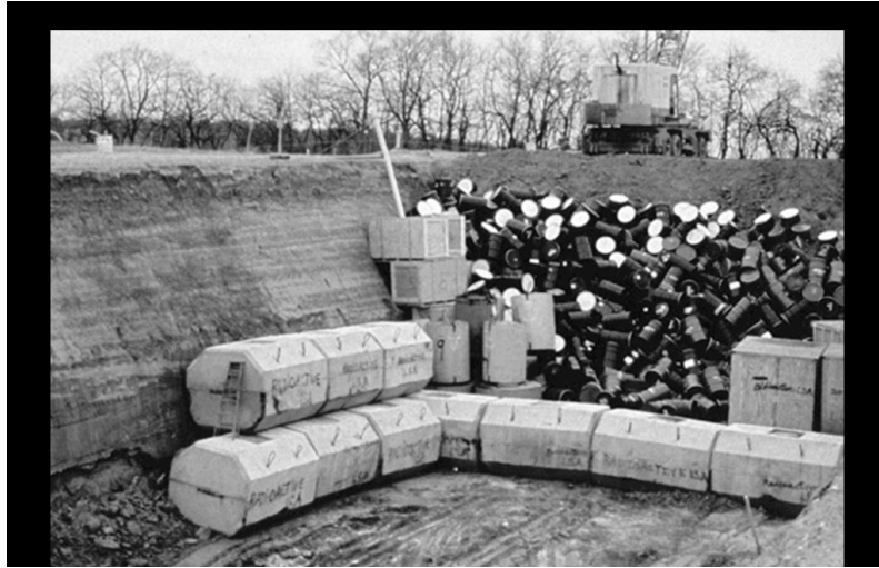
Photo 3 - Burial of LLRW at the Sheffield LLRW Disposal Facility (IEMA, date unknown)
