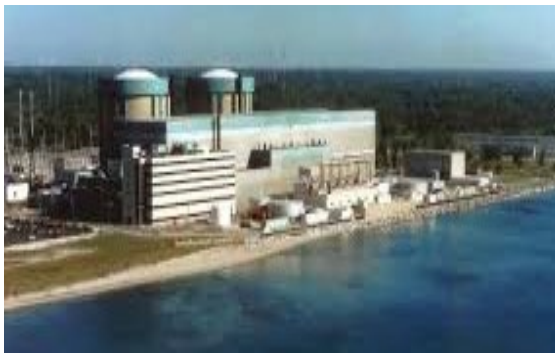
Zion station prior to decommissioning
