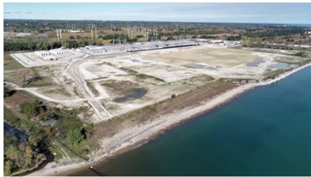
Zion station post building and equipment removal
