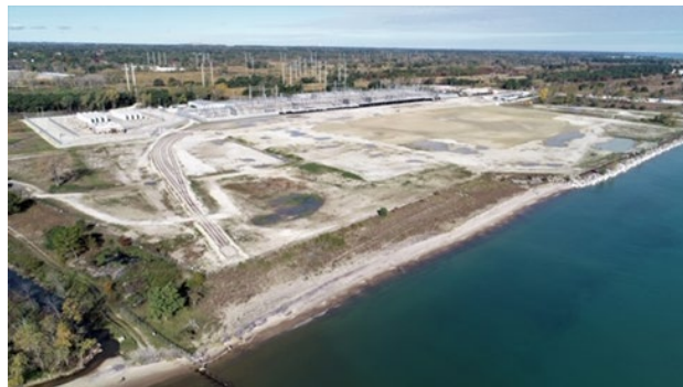
Zion station post building and equipment removal
