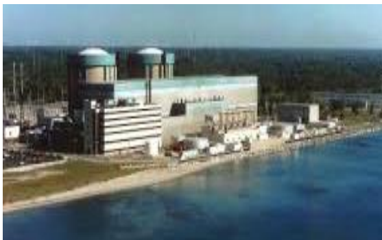
Zion station prior to decommissioning
