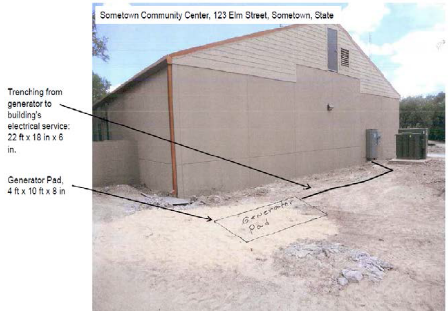
Figure 4. Ground-level photograph showing proposed ground disturbance area.
