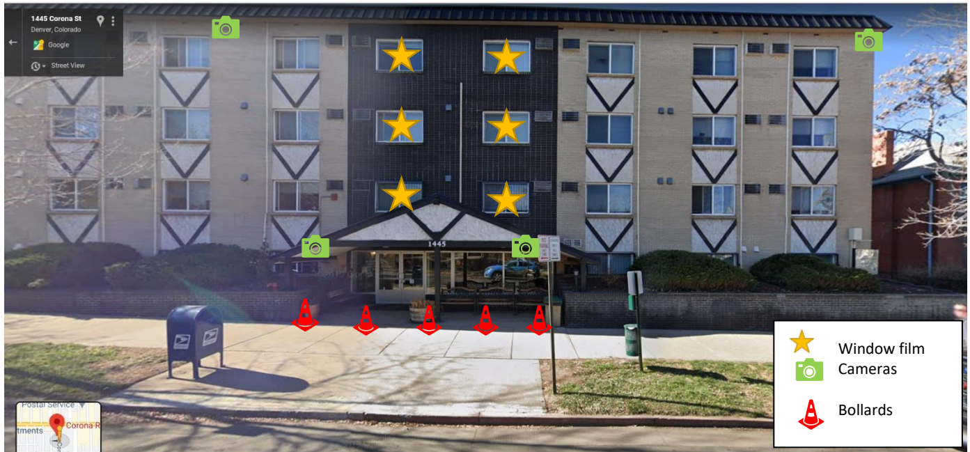
ground-level photo showing where installation will occur
